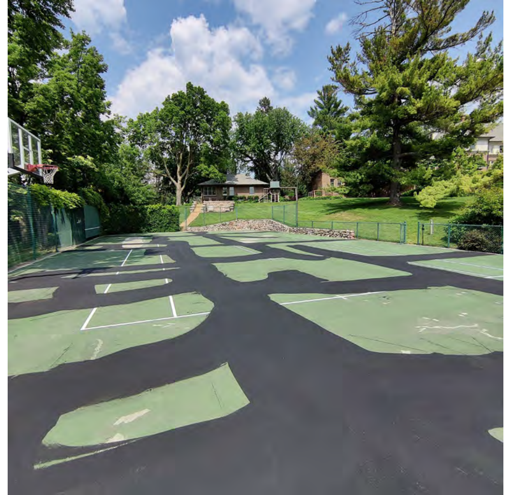
Coat with Acrylic Resurfacer
